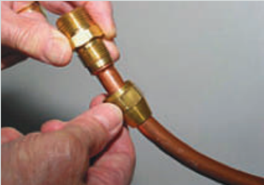
Figure 7.1a Assembling Copper Flare Pipe Adaptor and Nut
