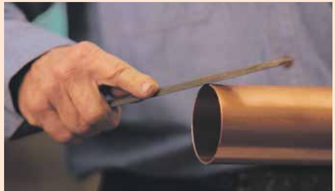
2. Carefully deburr and wipe clean the end of the tube internally and externally to minimise turbulence and pressure loss according to AS3500 and avoid damaging the O-ring.
