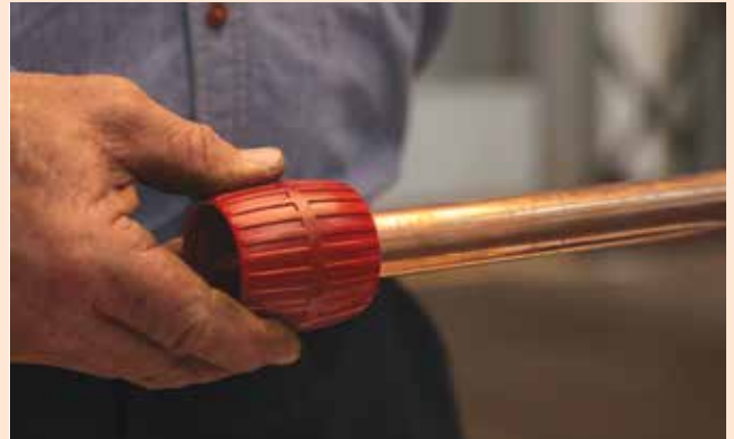
2. Deburr carefully the end of the tube on the inside to minimise turbulence and pressure loss according to AS3500 and on the outside to avoid damaging the O-ring.
