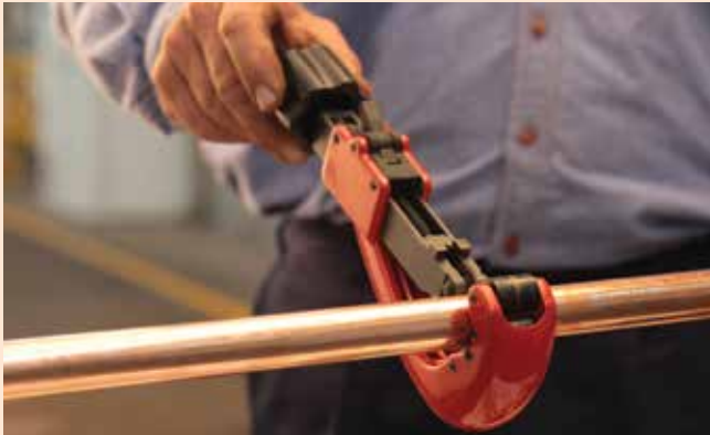
1. Cut copper tube to length using a pipe cutter.
