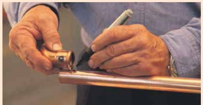
4. Mark the insertion depth by lining up the fitting side by side with the tube and mark the tube. When the fitting is inserted onto the tube the outer edge of the fitting must line up with the marking. For correct insertion depths see column e of the Fittings Space Requirements table, page 22.
