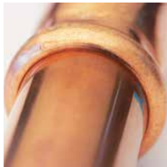
Pressed fitting - no gap between fitting and tube.
